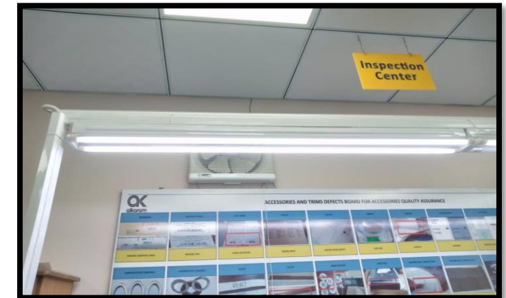
Installed LED (42W) Lights in AQA Department
